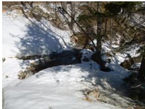
Snow covered downstream north and south embankments.
