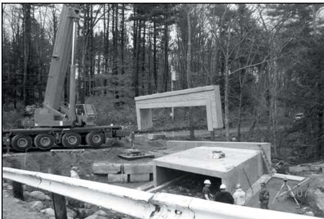
Bridge face being lowered at White Birch Point
